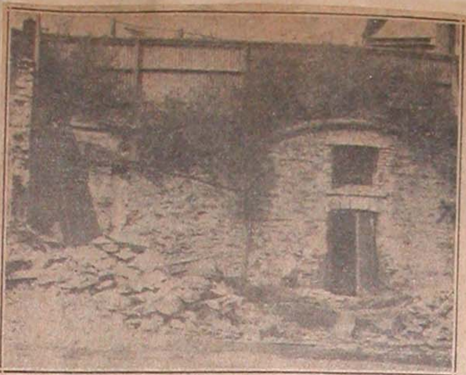
FROM PRISON TO TRANSFORMER STATION—Workmen are shown demolishing an old building north of Elder Conservatorium in the grounds of Adelaide University. In the early days it was used as a powder magazine, and for a time during the war when the Jubilee Oval was set aside for military purposes, it served as a military prison. The University then used it as an anatomical department. It will be replaced by a transformer station for the supply of electricity to the University and neighboring institutions.
