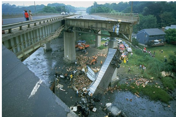
Figure 1. Collapse of Interstate 95 Mianus Bridge in Connecticut - USA (Kirk & Mallett 2007)
