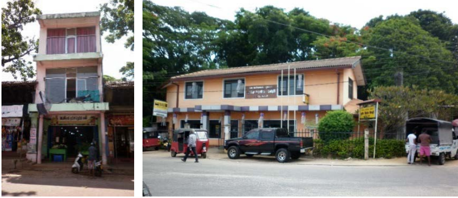
Digana- shop modified in to three storey pink building and the pink colour Bank building instead of white colour (MAU colour code).
