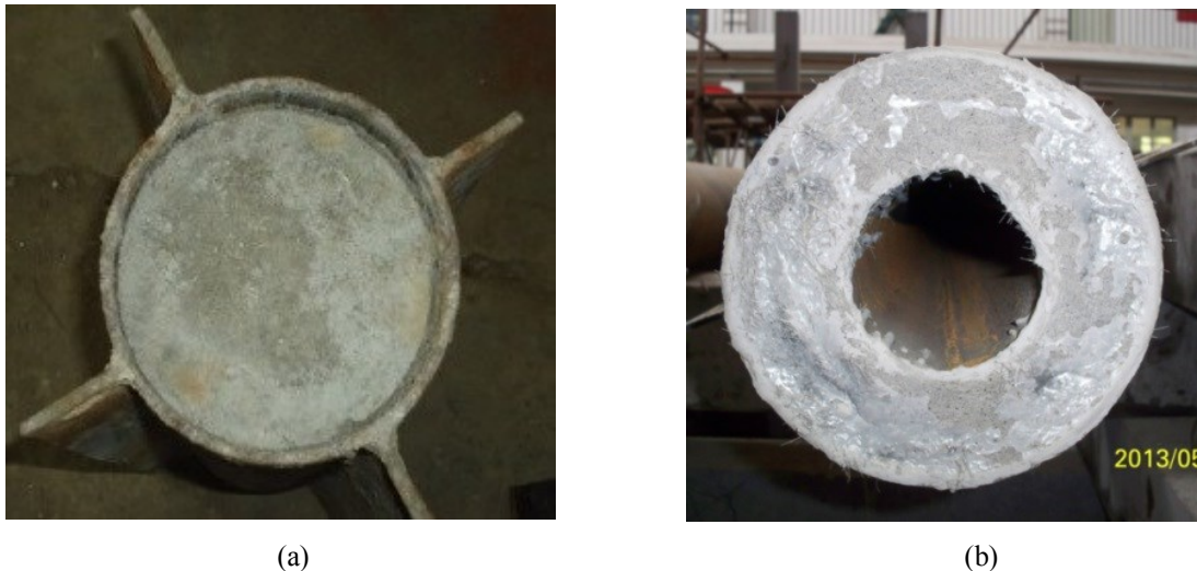
Fig. 1: The typical cross section of (a) a circular CFST (left) and (b) a circular CFDST (right)
