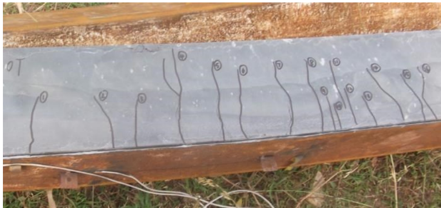
(b) Crack propagation in concrete
