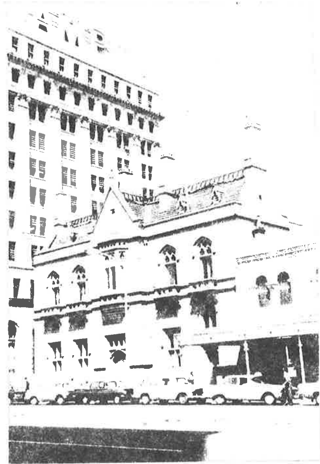
FIG.54 - E.S. & A. BANK INTIMATE LANDMARK
