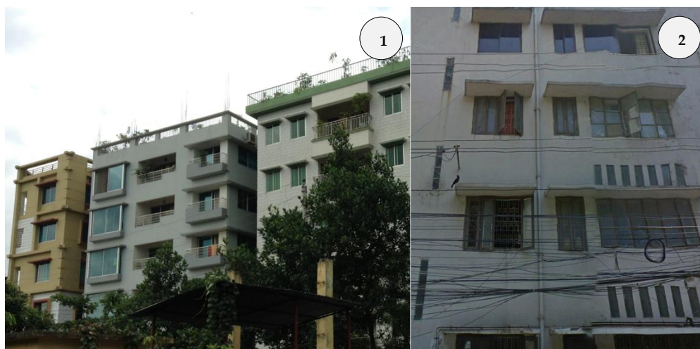
Figure 7.4: Examples of Aluminium Sliding and Shutter-type Windows. Source: Field Study (1), Google Earth (2)
