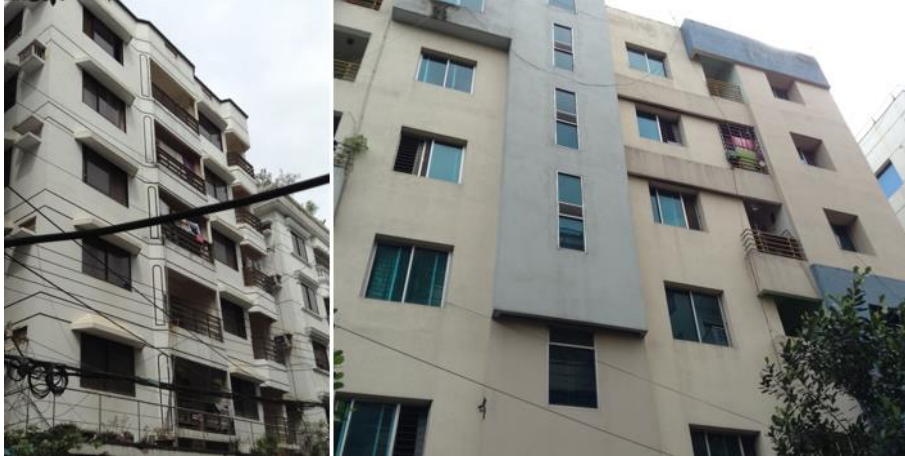
Figure 5.26: Examples of Horizontal Shading & Recessed Windows. Source: Field Study
