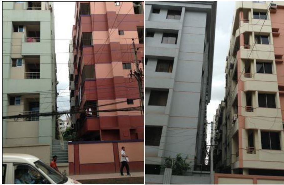
Figure 5.12: Distance Between Buildings at the Back. Source: Field Study
