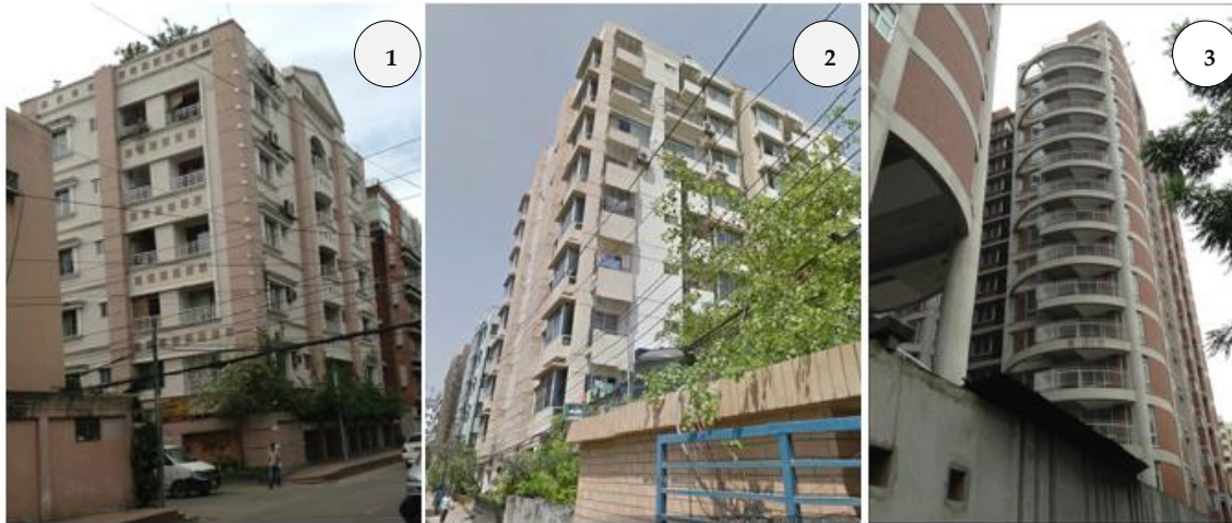
Figure 2.7: Examples of Walk-up, Mid-rise & High-rise Apartment Buildings. Source: Author(1,3) & Adapted from Google Earth(2).
