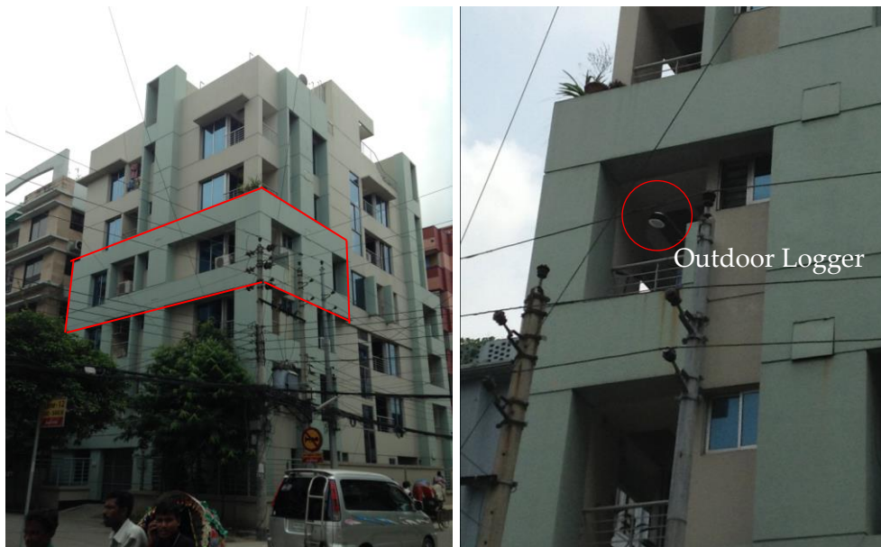
Figure 8.2: The Case Study Apartment and the Outdoor Logger
