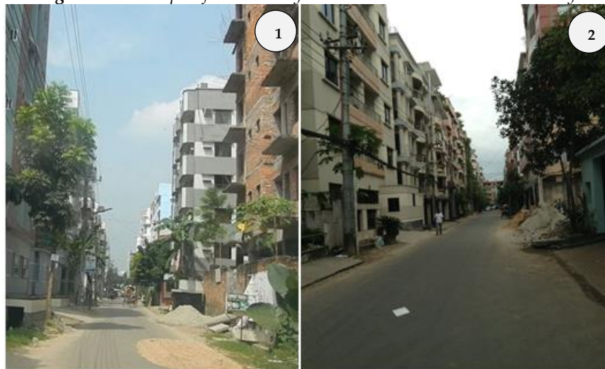
Figure 5.9: Examples of Access Roads in Uttara (1) & DOHS (2). Source: Field Study
