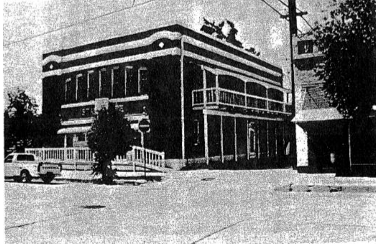
Figure 1. Gilroy Firehouse (Tena-Colunga & Abrams 1992)
