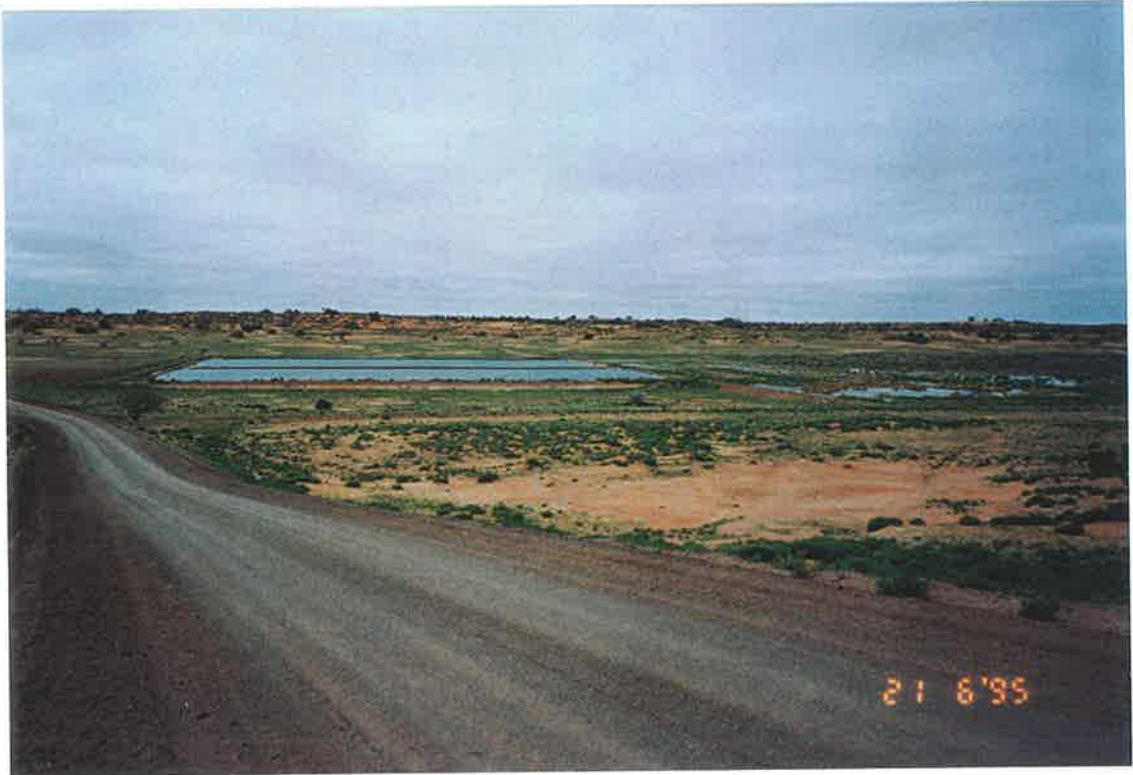
Plate 8.7: Evaporation ponds containing water brought up during mining of oil and gas.
