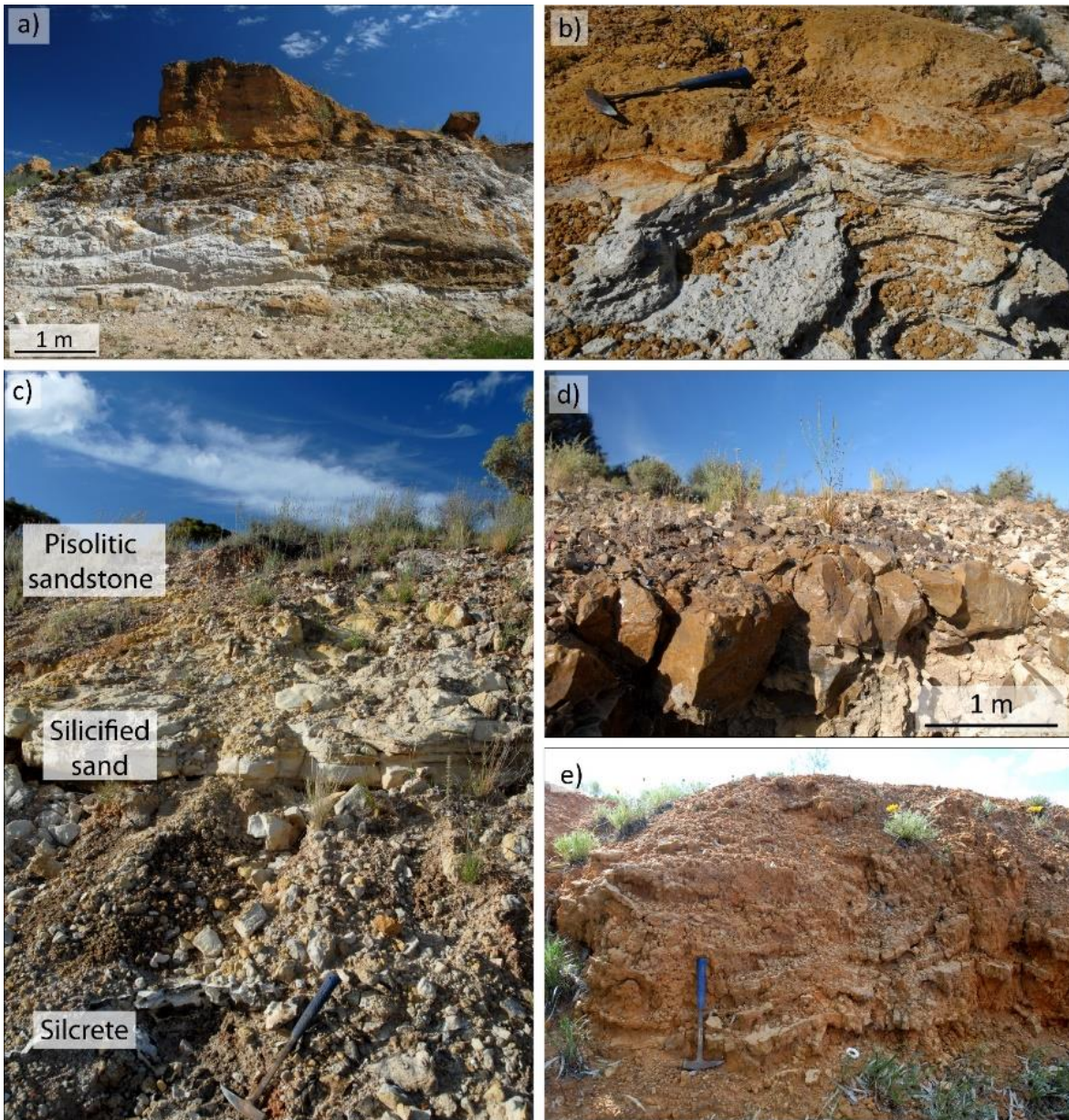
Figure 4.7 a) Profile of the Loxton-Parilla Sands at Ultima. Cross-bedded, muscovitic, fine sand is overlain by laminar silcrete, which is in turn overlain by mottled and pisolitic sandstone. The deep marks in the pale sand are scour marks from quarry machinery which obscure cross-bedding. Note the solution hollow that has been filled with transported material on right hand side of profile, b) which obscure cross-bedding. Note the solution hollow that has been filled with transported material on right hand side of profile, c) Indurated weathering profile of the Loxton-Parilla Sands exposed at Lyrup. Massive silcrete overlain by kaolin-rich sand, which is overlain by mottled and pisolitic sandstone. Hammer is 45 cm long, d) Massive jointed silcrete at Lyrup, e) Undulating silica hard bands at Nyah. Bands are fractured, forming silica-rich nodules. Hammer is 45 cm long.
