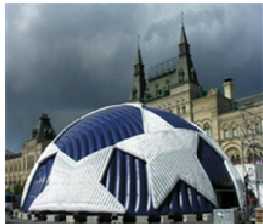
(b) Champions League Dome in Madrid: an example of a temporary membrane structure.
