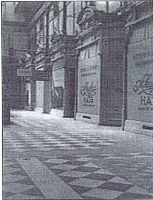
Figure 13 Photos were used to identify the original flooring and detailing. (MortlockB13364)
