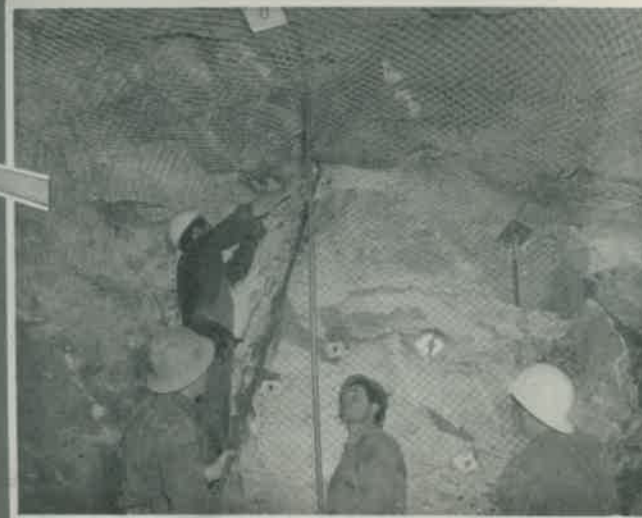
4 Placing of wire mesh on roof
