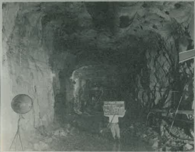
1 Excavation of centre drive
