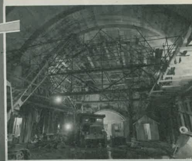
6 Placing of concrete arch ribs in roof
