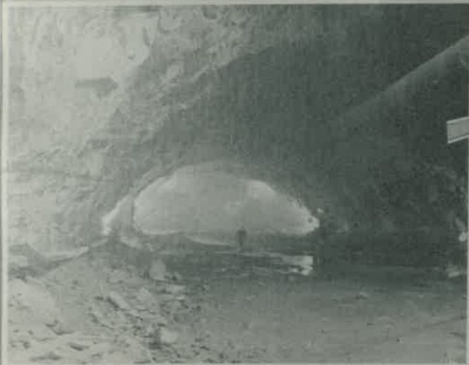
3 Completion of excavation of roof
