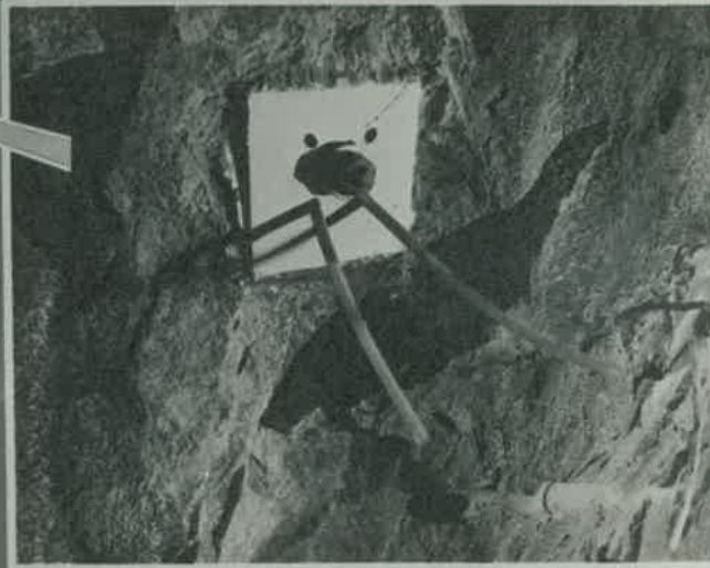
2 Installation and grouting of rock bolts
