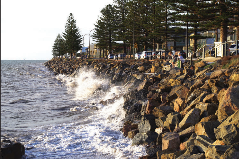
Figure 1.5 View north along the metropolitan coast during high-tide conditions at Brighton in 2014, showing rip-rap boulder protection of the coast. The rock wall is designed to absorb wave energy and allow water to percolate slowly back seawards without scouring the beach. The large facing boulders are progressively underlain by layers of smaller rocks, allowing penetration by water but not of the rocks themselves. Many sections of the metropolitan coast are protected in this way.
