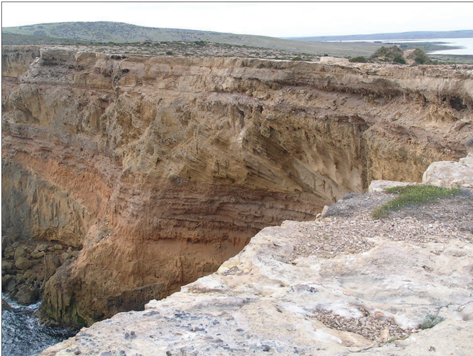
Figure 10.18 Narrow neck of land at Cummings Monument, separating the ocean from Lake Hamilton in the background. Note the cross-bedding in the aeolianite cliff, the fossil soils and the calcreted upper surface. The cliff is about 50 m high.
