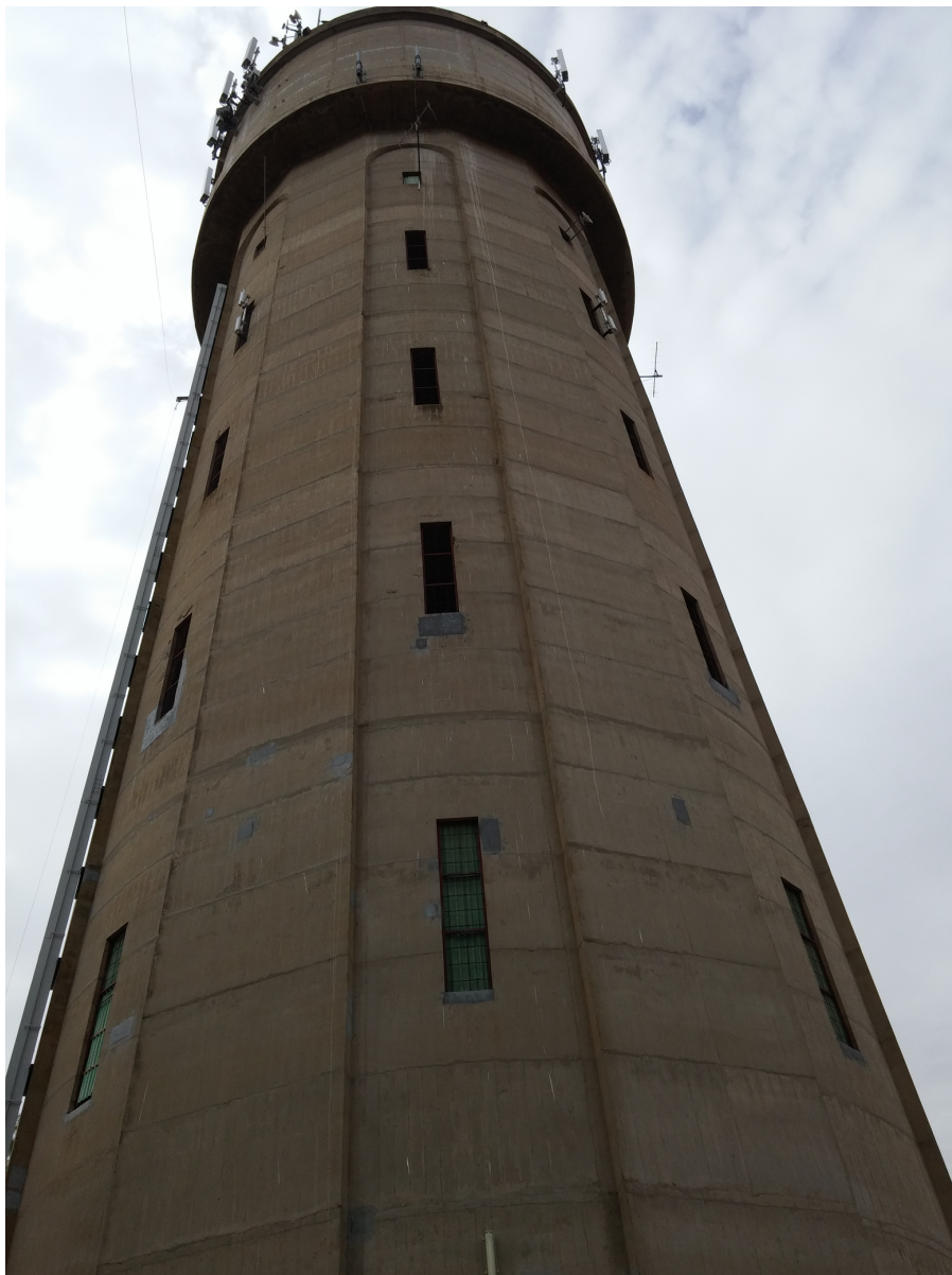
Figure 4-6: Ground view of the 50 metre tower where the repeater antennas are installed. Antennas are positioned on the top floor's windows and are separated by the concrete structure with two windows between them.
