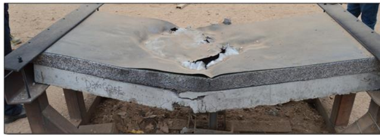
(a). Foam-protected RC slab after explosion
