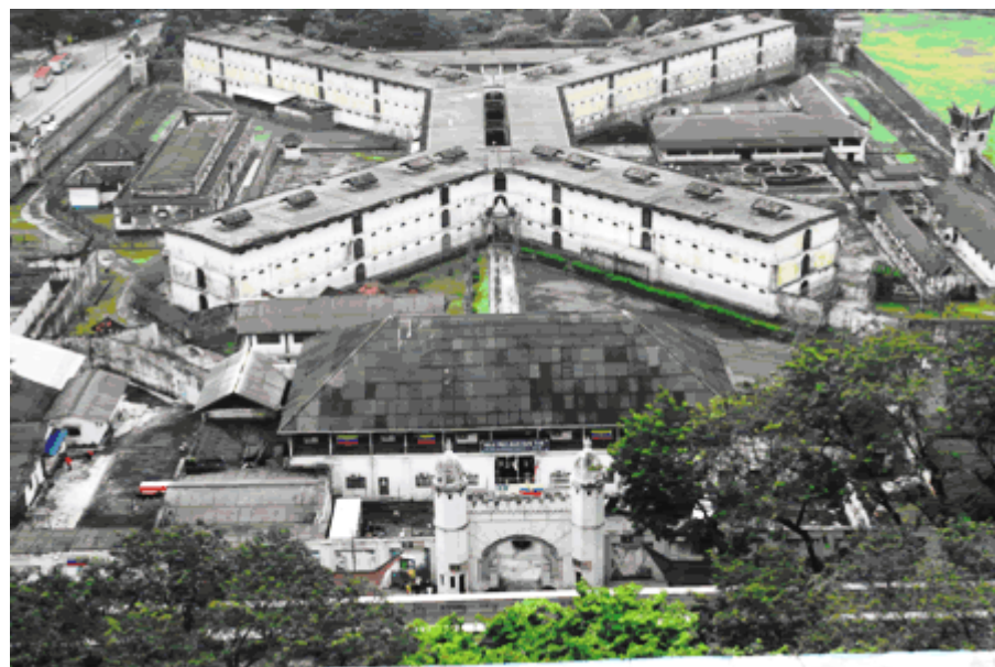
Figure 2.20: The X shape plan of the Pudu Jail is said to be similar to Kindy Jail, in Bogambia. Source: (Jabatan Penjara Malaysia, 2008).
