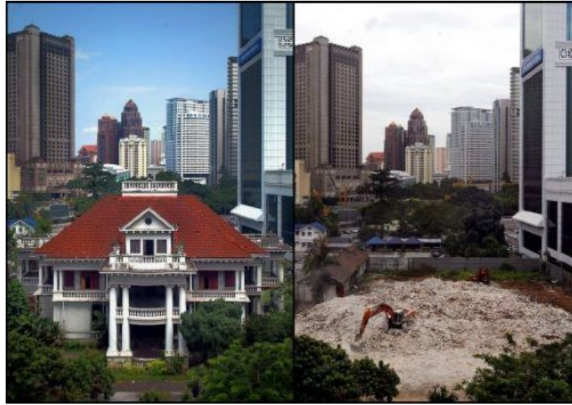
Figure 2.19 (a) The Bok House before demolition; (b) after the demolition process. Source: (The Star, 2006).
