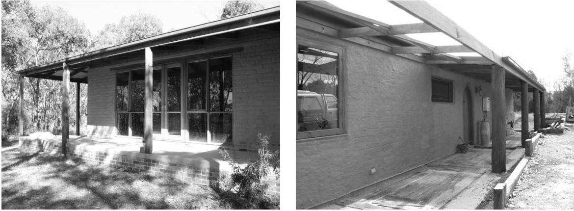
Figure 5.4. More contemporary examples of earth construction; left house built in 2001 & right house built in 2010, Melbourne
