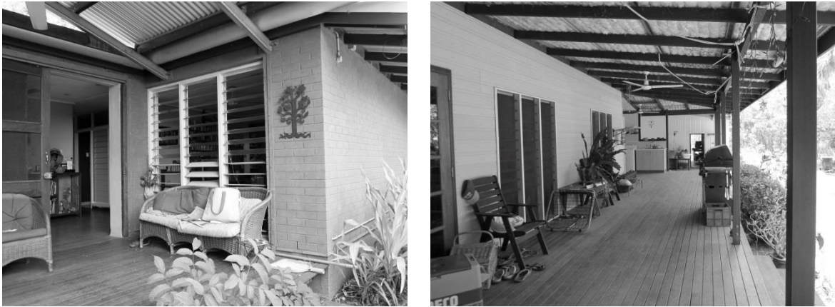
Figure 5.5. Left image, an example of heavyweight construction & right image, an example of light weight construction, Darwin
