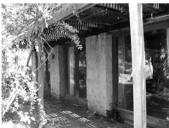
Figure 5.3. Post and beam construction with mud brick infill predominantly used in Melbourne houses
