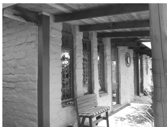
Figure 5.3. Post and beam construction with mud brick infill predominantly used in Melbourne houses
