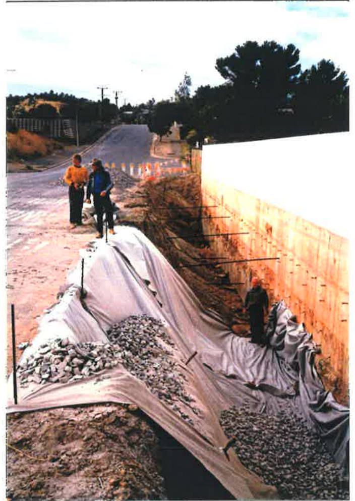
(b) during placement of the backfill
