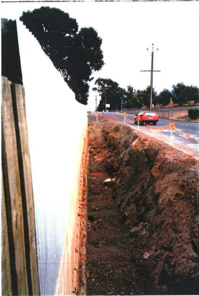
(a) before placement of the backfill
