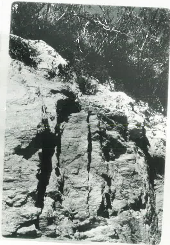
PLATE LV. Typical jointing in the Warren Schist, outcropping along the pipeline track west of the Warren Reservoir.
