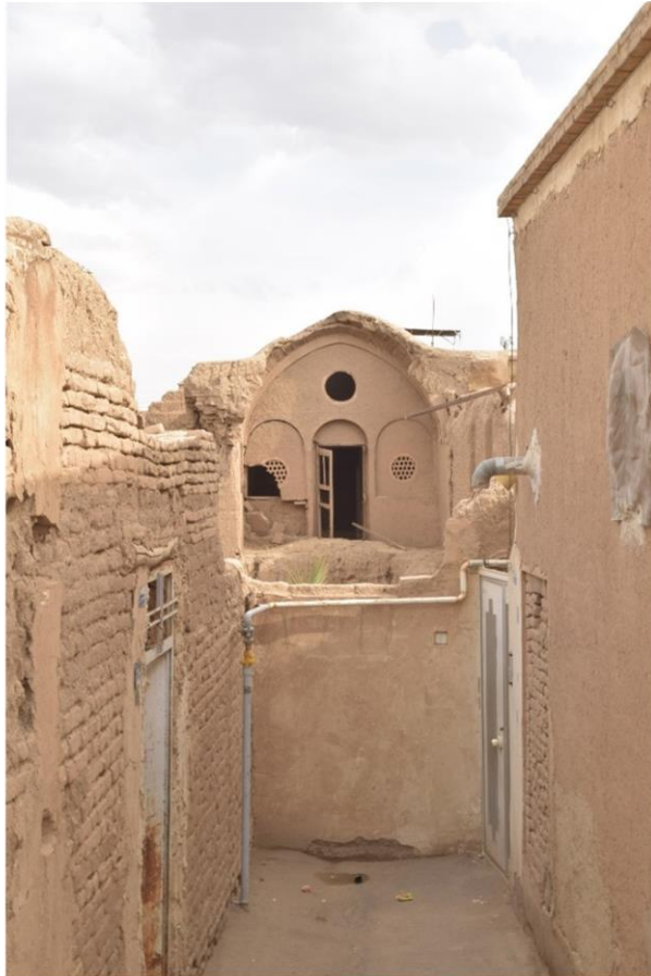
Dilapidated abandoned urban fabrics in Kashan, 2018 (Source: author)
