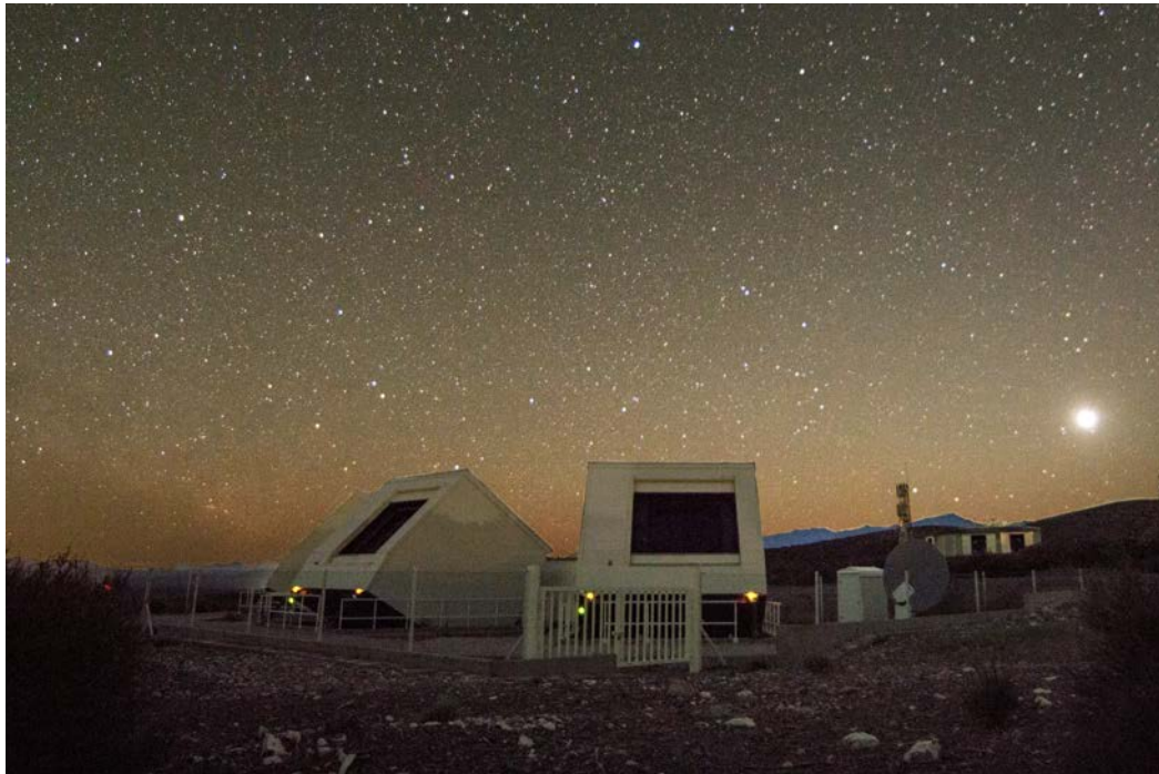
Fig. 2.28. HEAT in operation. (Image by the author).
