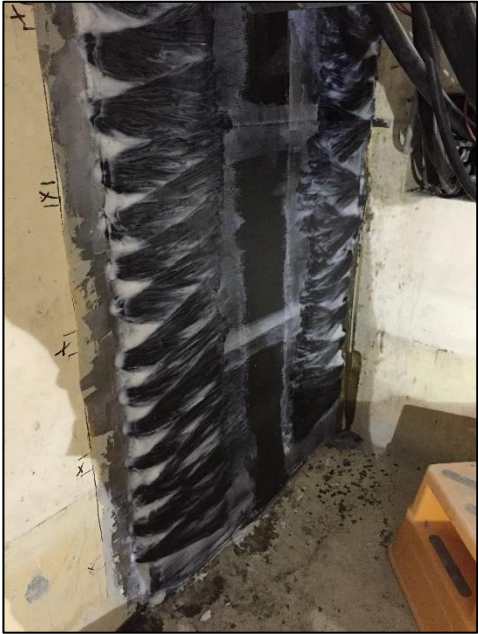
(b) Example of using FRP anchors to close the confinement and bypass obstructions
