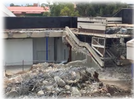
Figure 1.1: Example of construction and demolition waste (Photo taken by the author in Adelaide, 13/02/2018)
