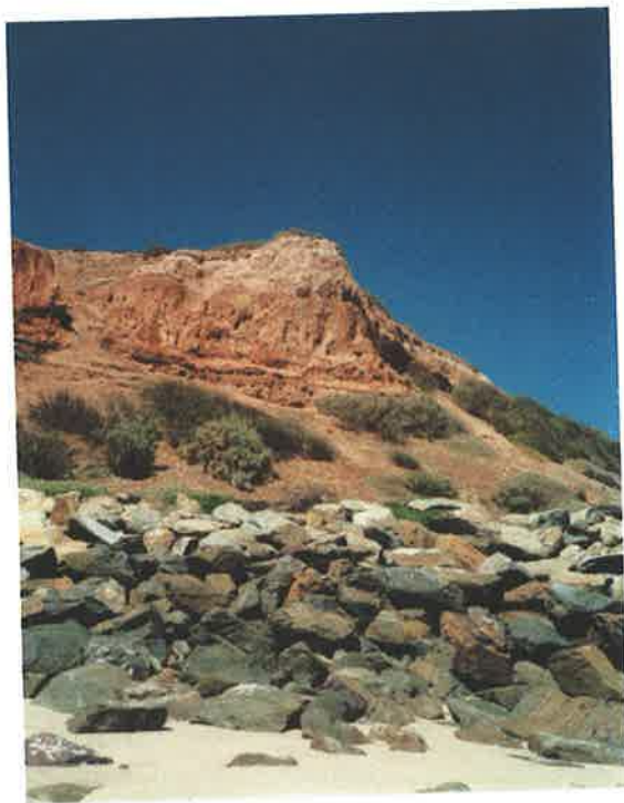
Plate 3.11 Witton Bluff is located by climbing down a man-made boulder retaining wall (shown in the foreground of this plate). A steep cliff comprised of a mix of clay and sand sediment, reinforced by the retaining wall, flanks the landward edge of this reef.
