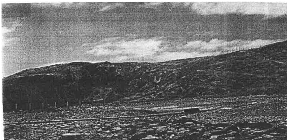
Plate A.1 The position of the Mitsubishi stormwater outfall and Mobil's treated effluent outfall adjacent to the northern refinery boundary (marked by the fence). The effluent pipe is in the foreground of the plate and the stormwater outfall pipe can be seen on the rising edge of the cliff in the background.
