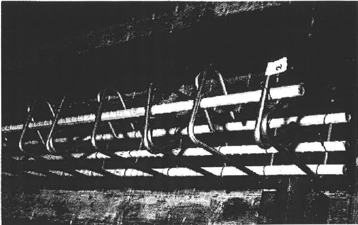
Figure 7.5. – Aerial view of the reinforcement cage of beam 2.
