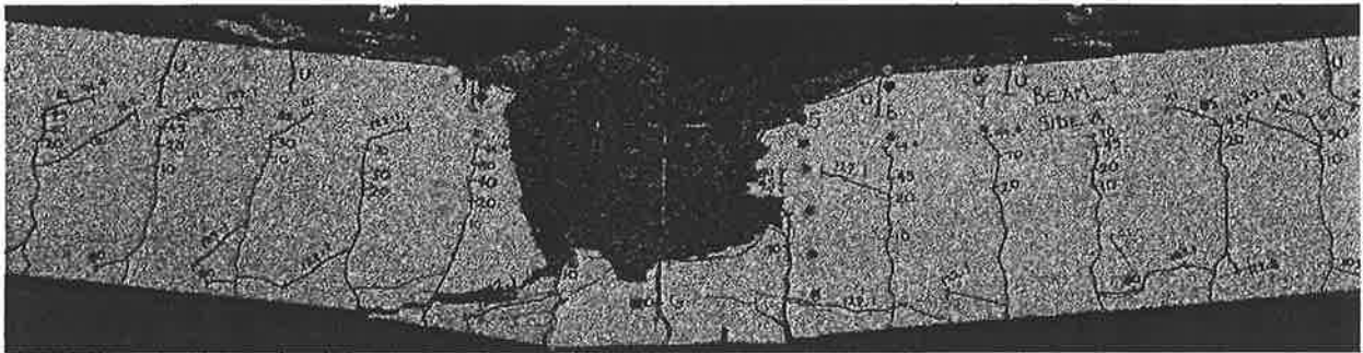
Figure 8.21. – Beam at failure.
