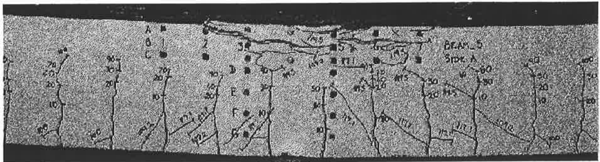
Figure 8.112. – Beam 5 at 119.5 kN.
