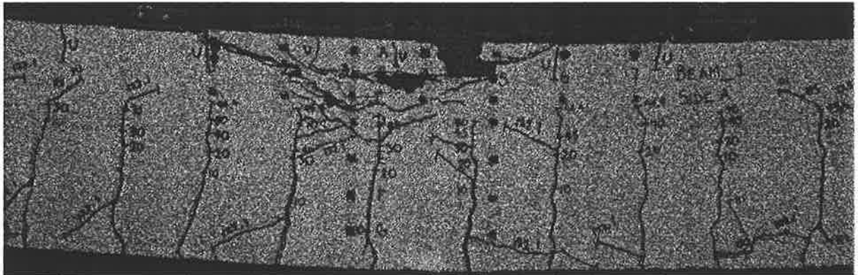
Figure 8.18. – Beam 1 at 122.1 kN.
