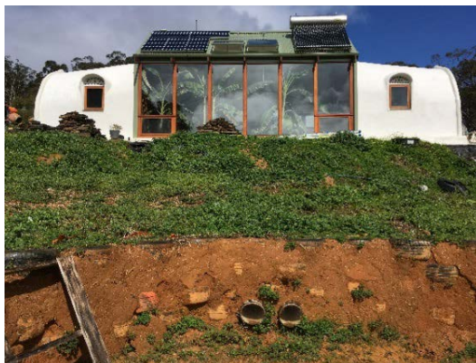
Figure 1: Earthship Ironbank (Note: earth tube inlets at bottom, centre of photo)
