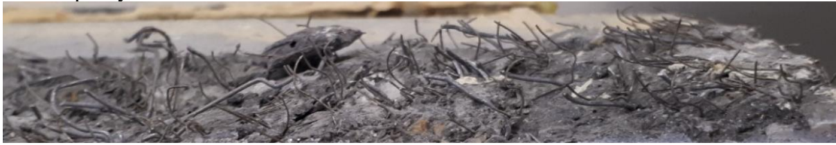
Fig. 11 Fibres at shear crack
