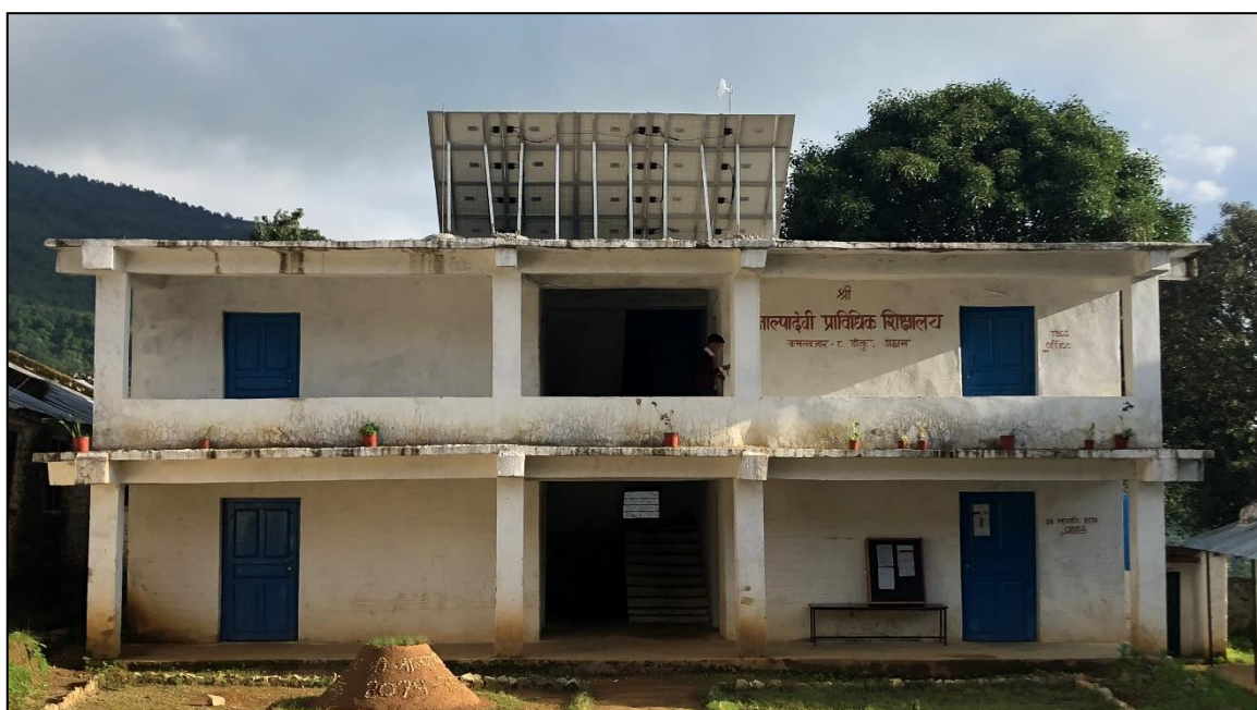
Figure 7.11 Solar PV panels on top of a school conducting ‘Junior Agriculture Technician’ course in Kamal Bazaar
