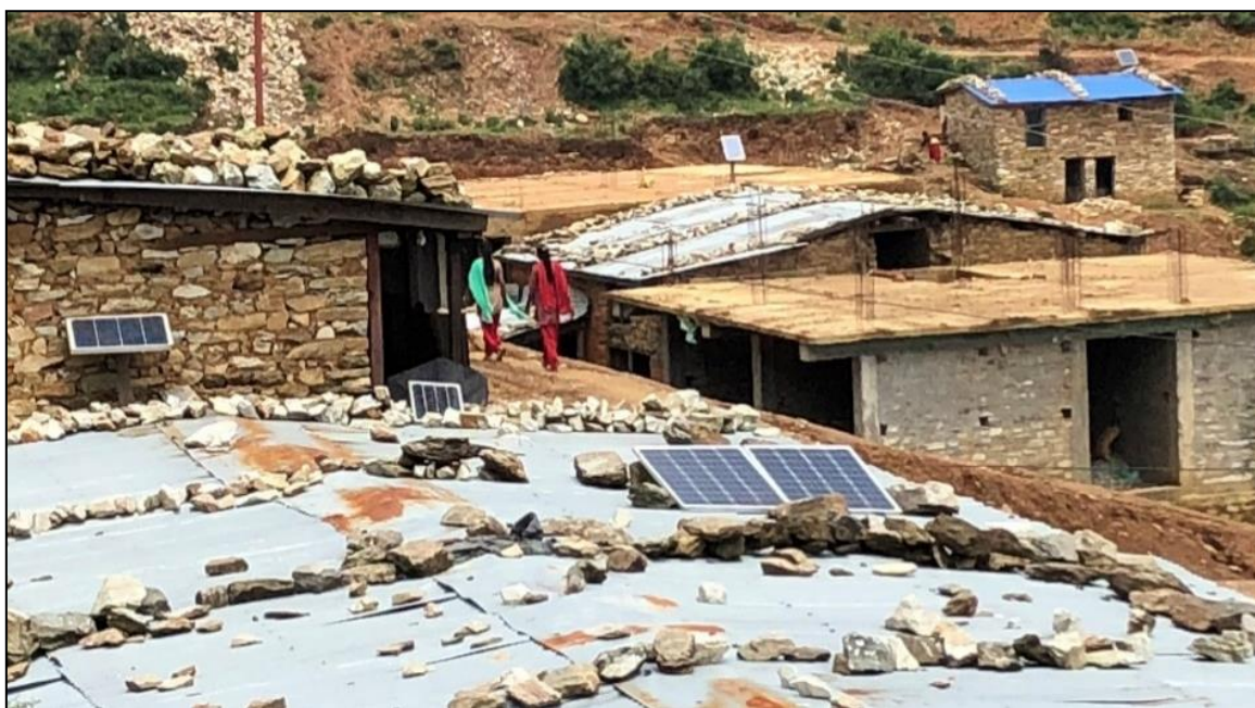
Figure 6.1 Solar PV panels on rooftops in Kama Bazaar, Achham
