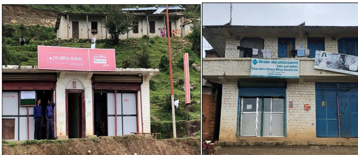
Figure 7.30 The bank (left) and the micro-finance business (right) in Kamal Bazaar get electricity from solar PVs and solar-wind micro grid for their operation
