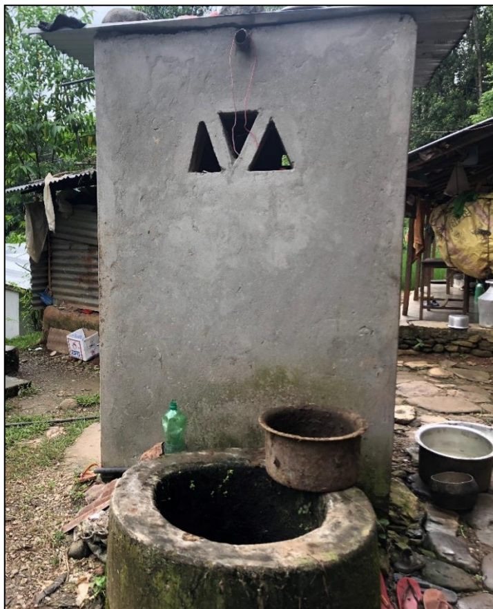
Figure 7.21 A ‘Pukka’ toilet adjacent to a biogas plant in Sunder Bazaar
