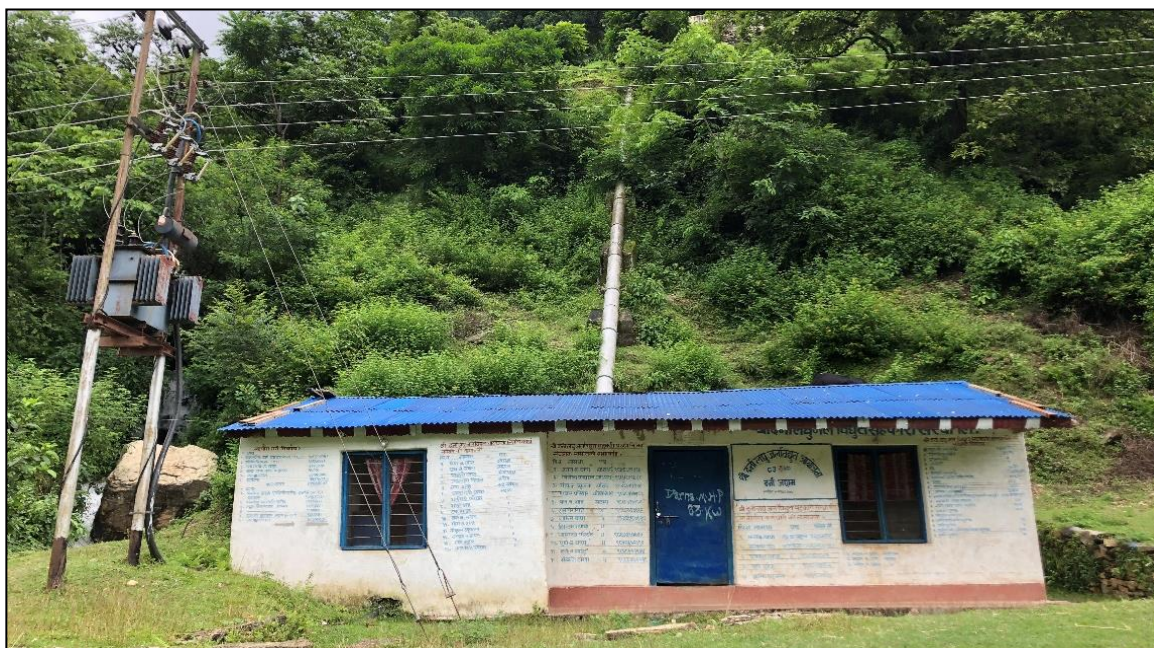
Figure 6.6 Micro-hydro powerhouse in Darna, Achham
