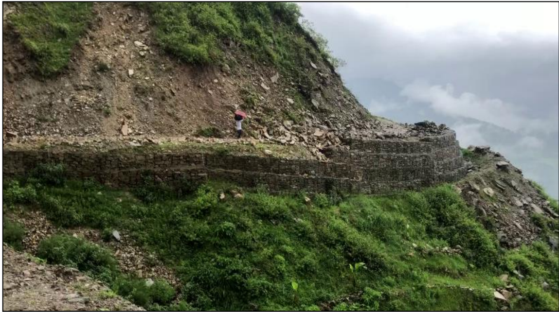
Figure 5.26 Roadside infrastructure to prevent landslides in Darna
