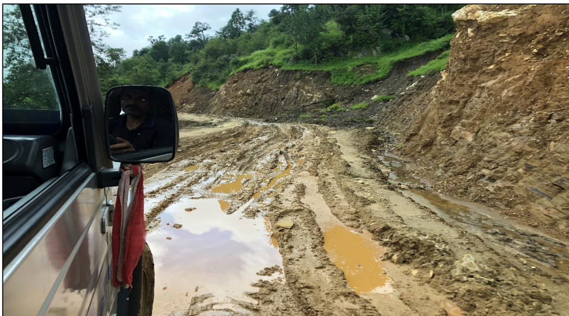
Figure 4.9 Dirt road at the onset of rainy season in Kamal Bazaar
