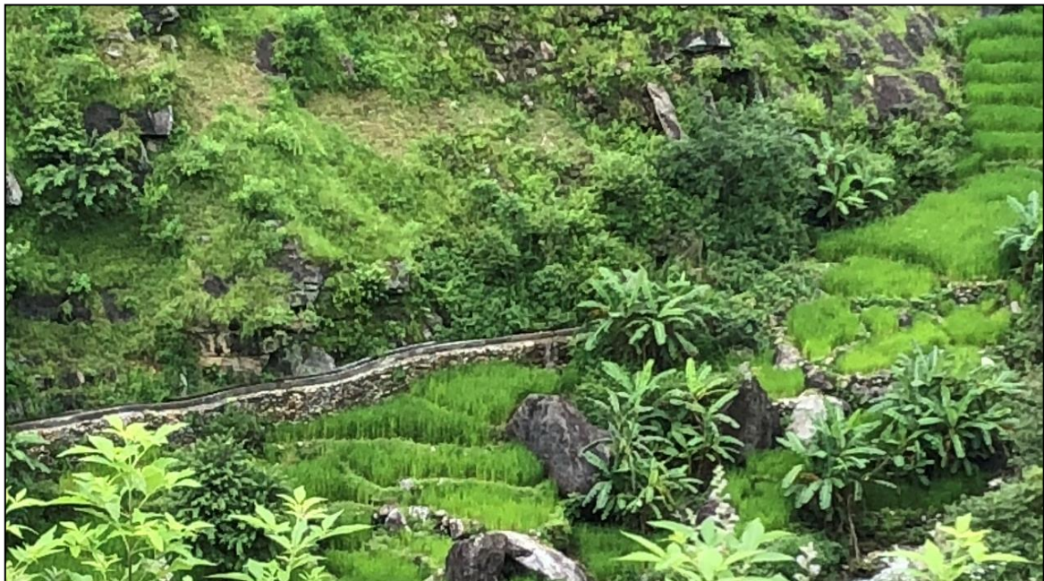
Figure 7.5 Micro-hydro facilitated irrigation infrastructure in Darna
