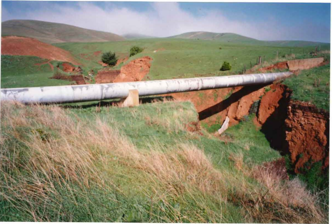
Plate 6b: The Myponga-Adelaide pipeline at Site A. Source: author.
