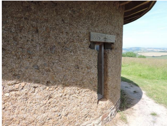
76 77 Figure 1. Exposed cob construction in Totnes, UK. 78
