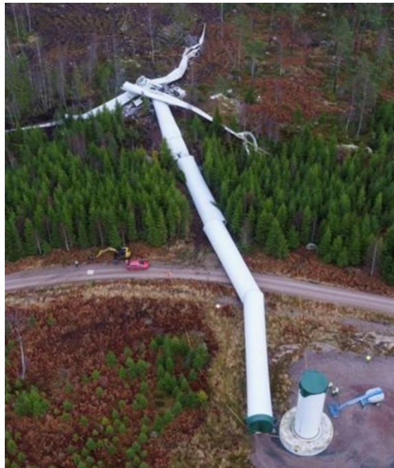
Figure 1. Vestas wind turbine collapse in Sweden [2]
