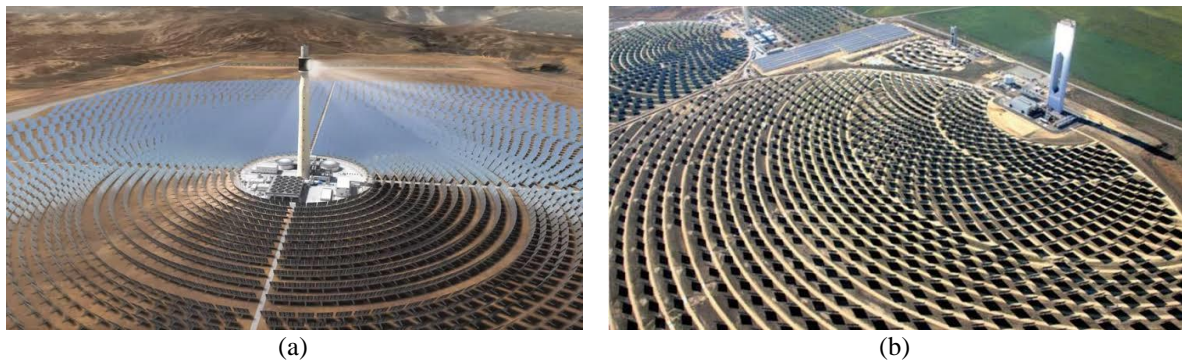
764 Figure 22. Different layouts of a heliostat field. (a) A radial heliostat field, Noor III in Morocco. Image from 765 www.masen.ma , (b) a polar heliostat field, PS10 in Spain. Image from www.eusolaris.eu .
