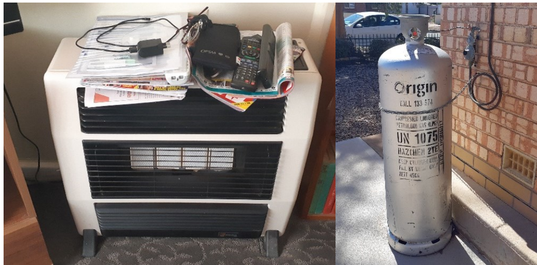
Figure 8-7 - House 53's LPG heater and LPG tank. Source: Photographed by the author
