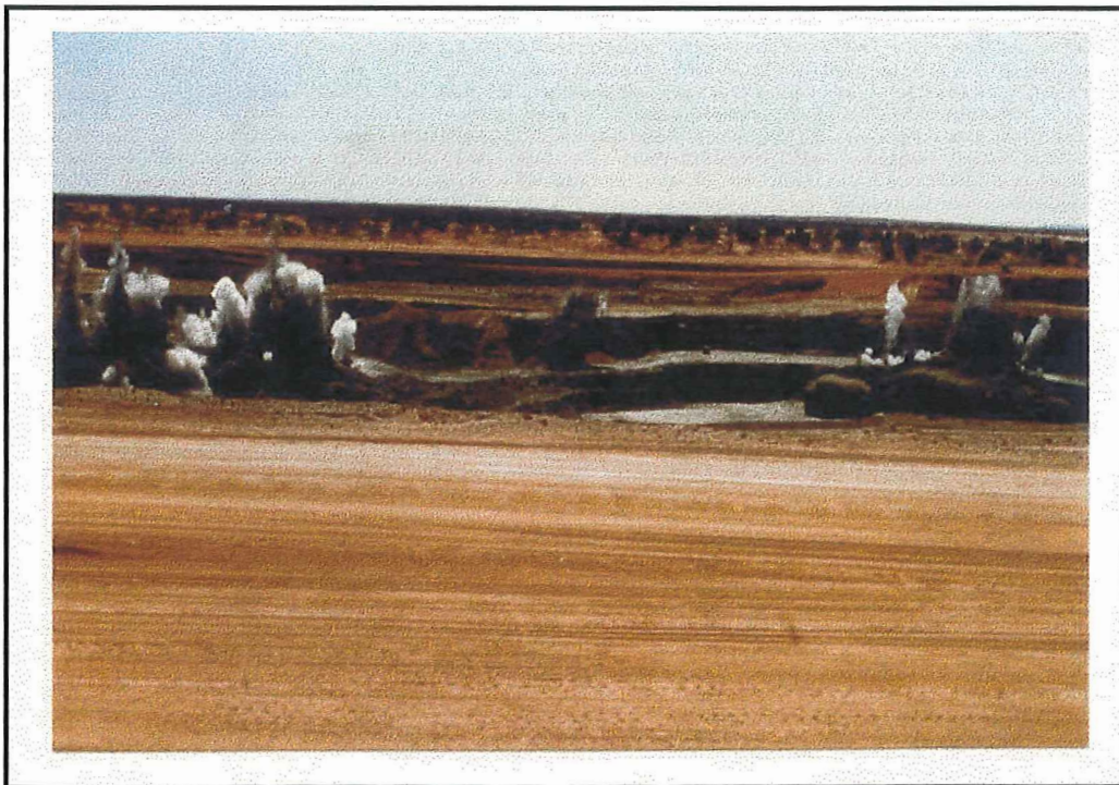
Figure 6. Blasting of the ore in the Cattle Grid open cut deposit (after CSR annual report 1974 – 1984).
