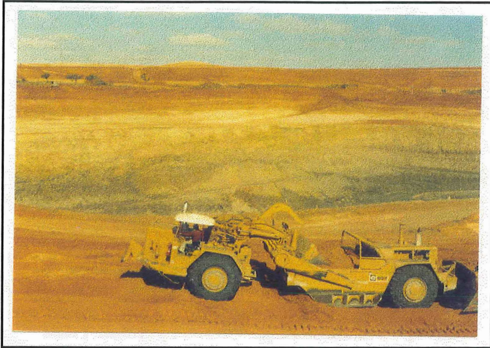
Figure 5. Removal of the overburden using heavy machinery (after CSR annual report 1974 – 1984).
