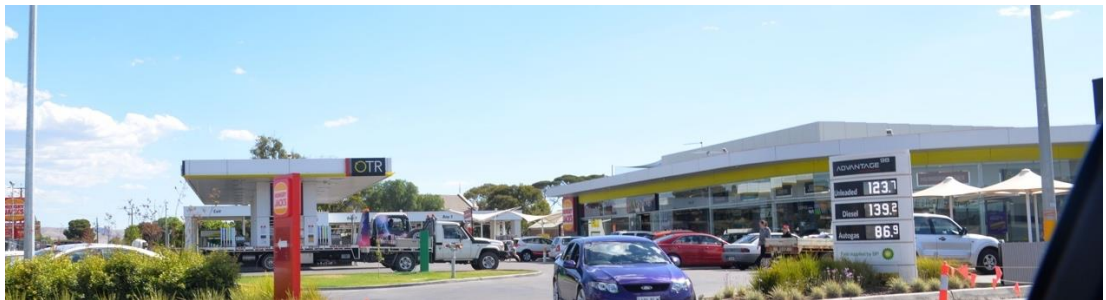
Figure 7.28: OTR fuel station view from South road (Source: author)
