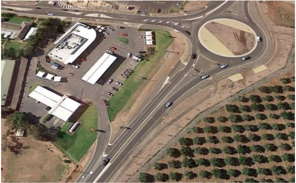
Figure 7.27: OTR fuel station (Source: Google Maps)
