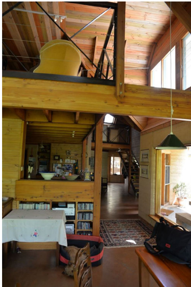
Figure 7.12: Interiors of one of the house, WGV, rammed earth wall, terracotta floor and timber frames (Source: author)
