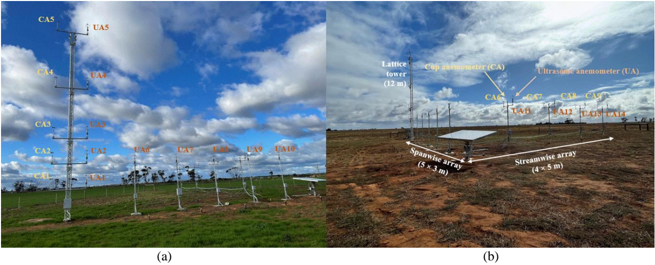
Figure 3. Completed installation of lattice tower, streamwise and spanwise mast arrays and instrumentation including ultrasonic anemometers (UA), cup anemometers (CA) and heliostat model at the ABLRF: (a) view looking north-east, (b) view looking north-west.
