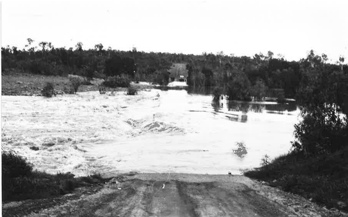
Figure 5.5: The Burketown crossing at Borroloola after a storm, January 1984
