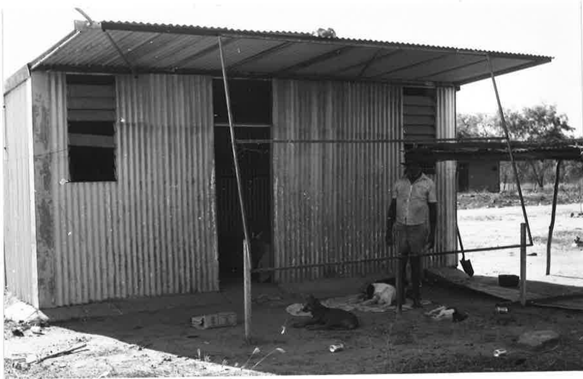
Figure 1.5: Typical old style iron hut
