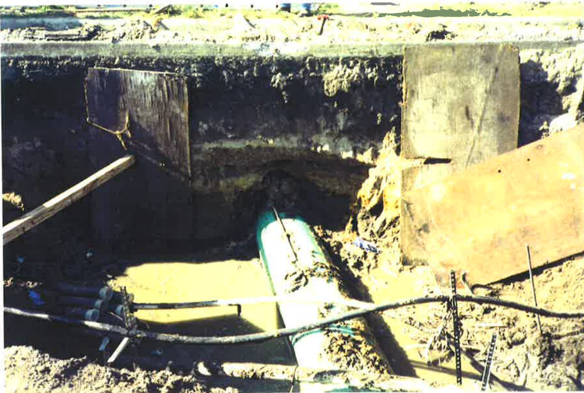
Figure C13: A boring operation underneath a road.
