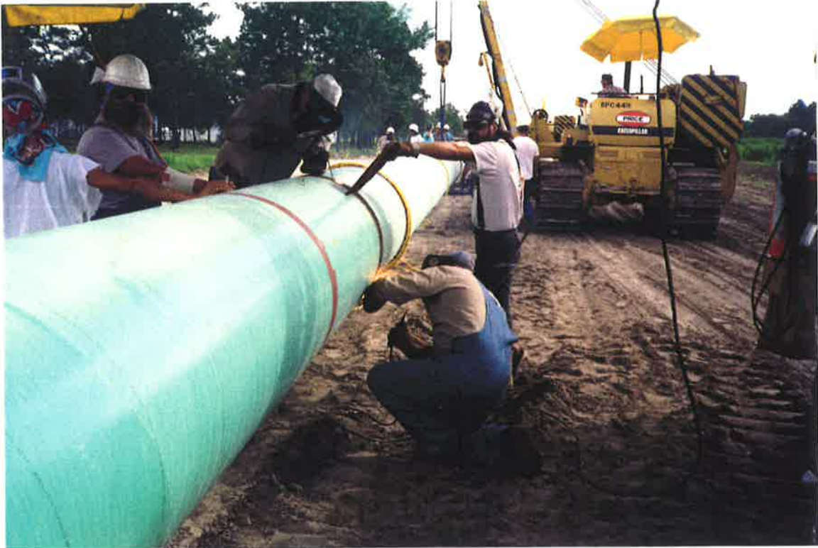
Figure C15: Welding of the root pass on Spread 8.
