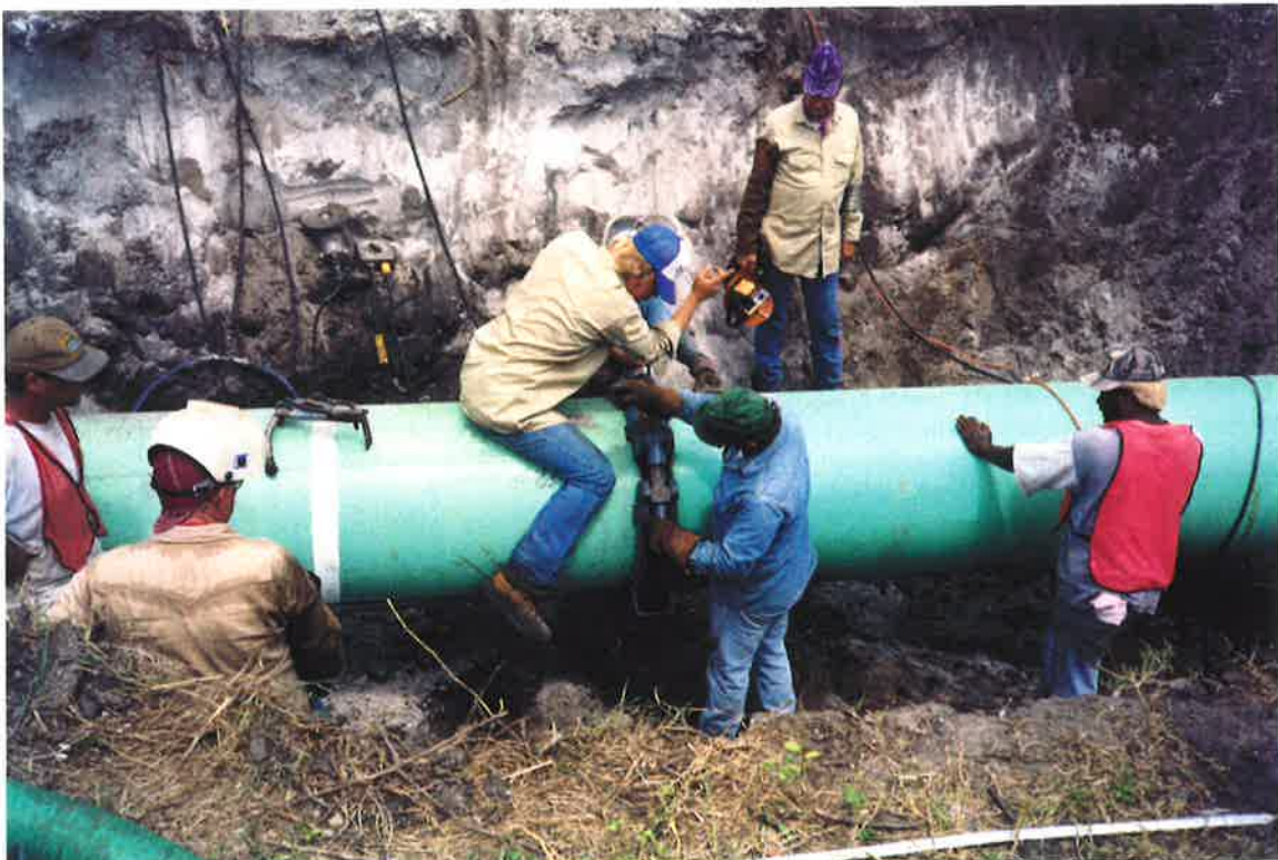
Figure C16: Preparation for a tie-in weld.
