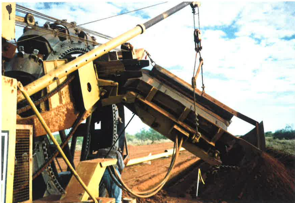
Figure C5: Photograph showing the trench being dug.
