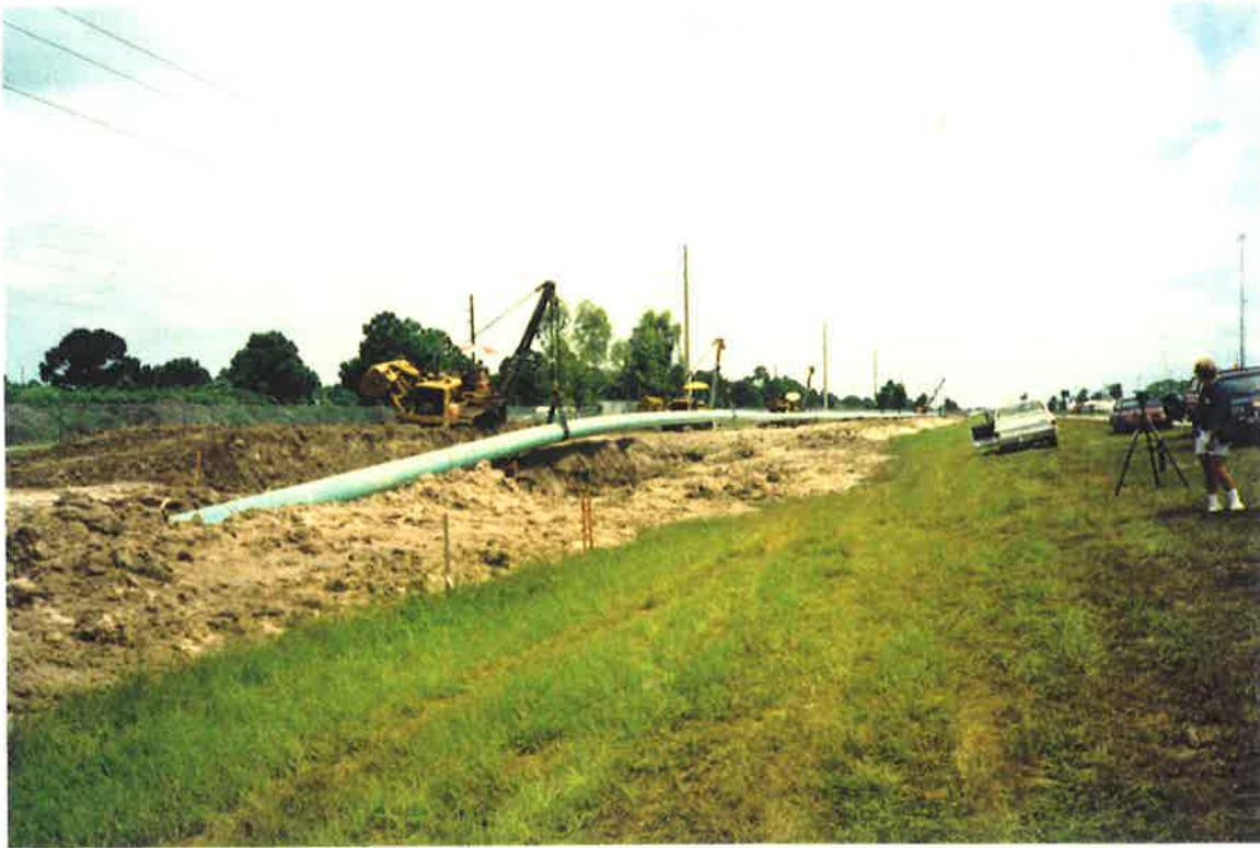
Figure C17: The lowering-in process of a pipe string.
