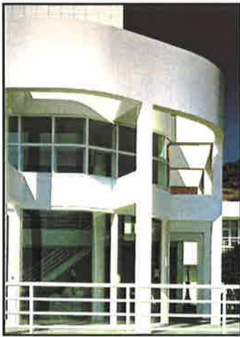
Fig. 3.27 Richard Meier. 1984-6. Ackerberg House , Malibu. South East corner Facade.
