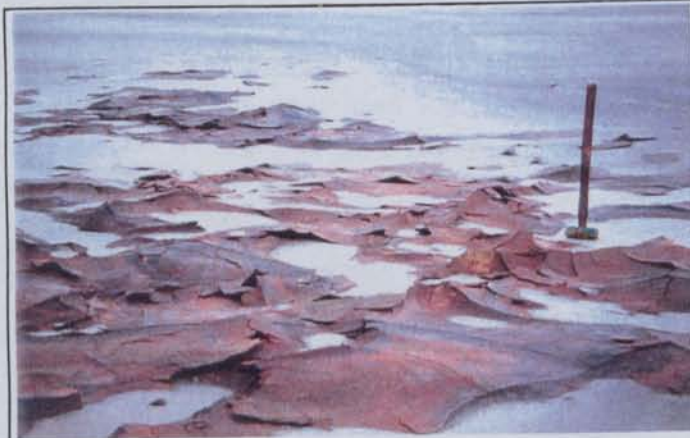
Photo 4.40 Blistered hardpan surface, Renison Bell, Dam C, Site 1
