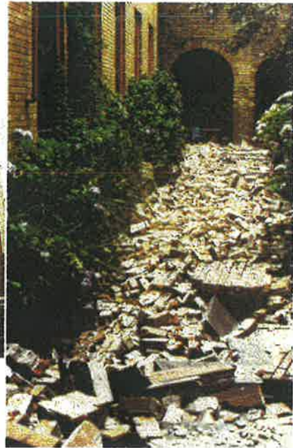
Figure 2.4.2 Parapet Failure, Tighes Hill Campus, Newcastle Technical College
