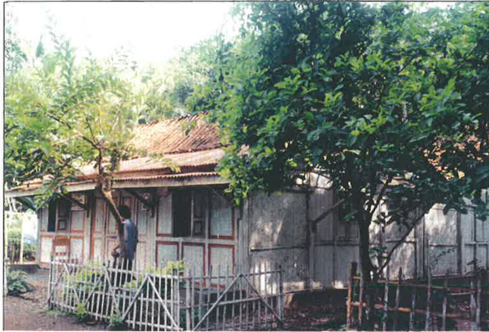
Plate 5. 9. A traditional Javanese house made of plaited bamboo combined with wood walls.
