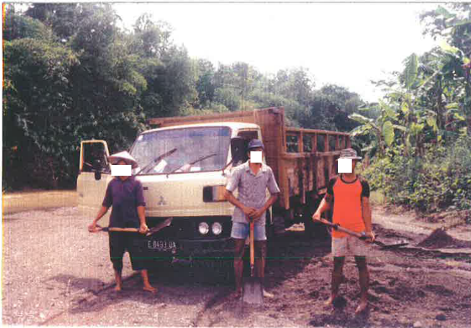
Plate 5. 3. Local sand gatherers are loading sand into a truck owned by a building material shop in Gombong.
