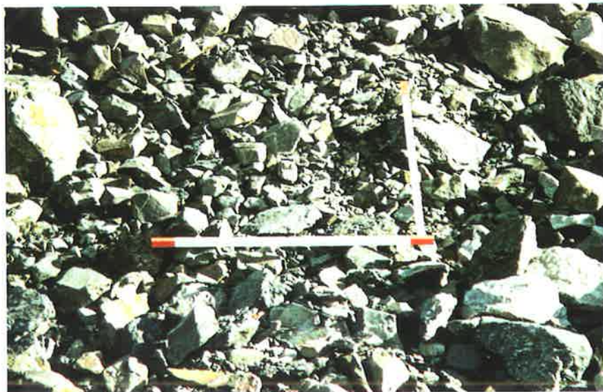
Plate 3-2 Close Distance Photograph of Dump Slope (Site 6)
