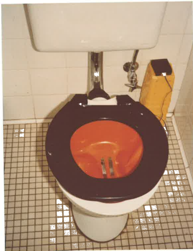
PLATE 5.2. The toilet alarm and bowl in place in the toilet.
