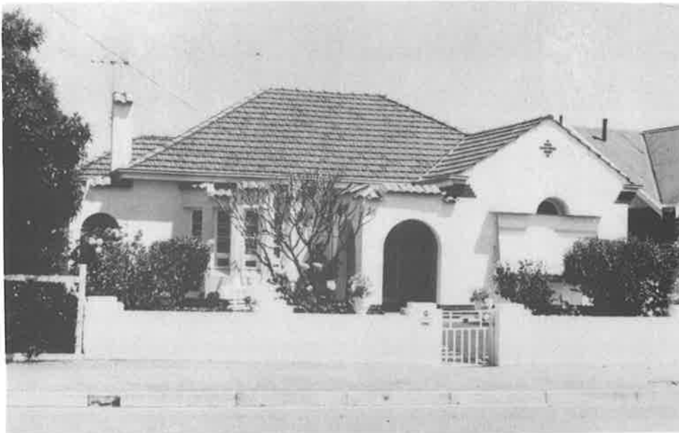
Plate 4.08. Spanish Mission, built 1935, Clarence Park; red brick walls with stucco finish, tiled roof.
