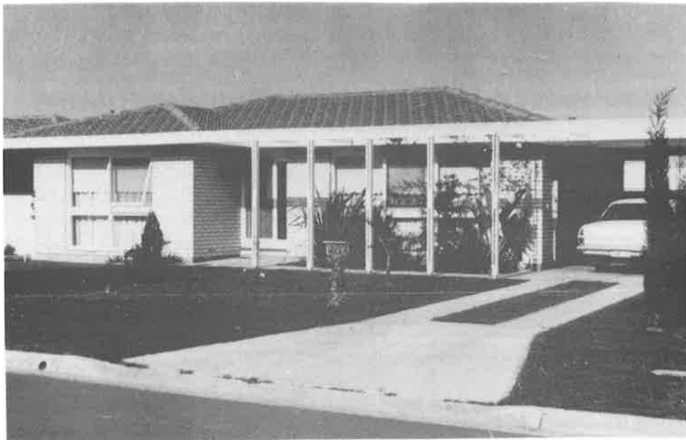
Plate 6.01. Pergola on Salisbury East house, connecting carport to front entry; of limited shading value until covered with vegetation.
