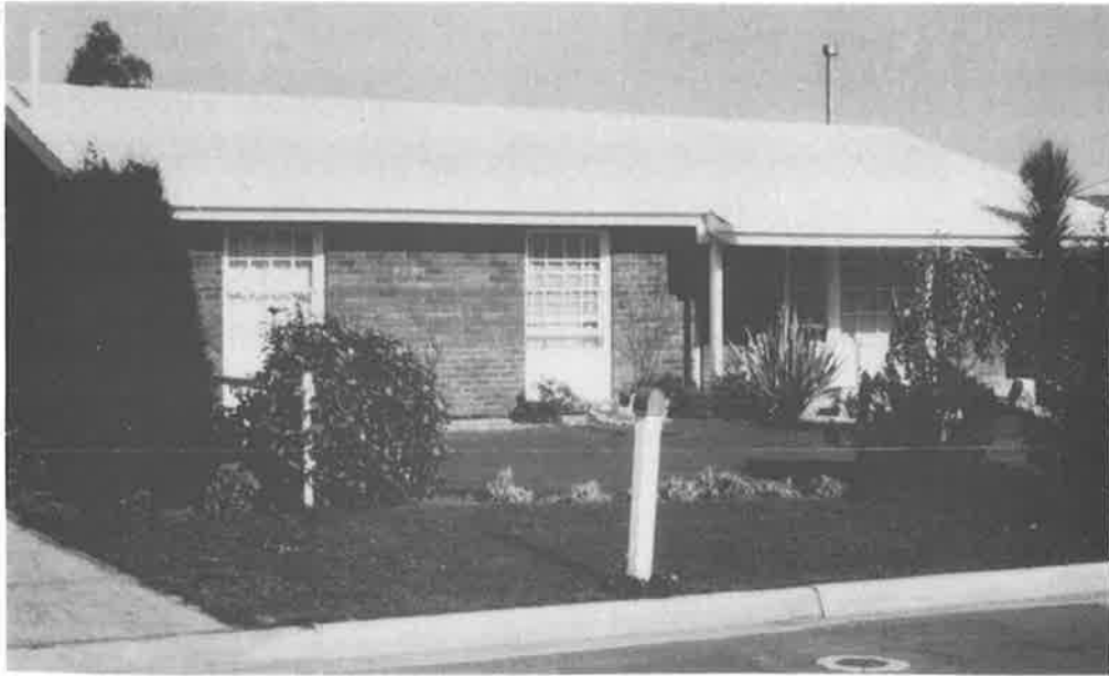
Plate 4.13. Colonial, built 1972, Salisbury East, red brick veneer walls, white tiled roof.
