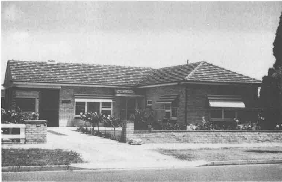
Plate 4.11. L-shape, built 1959, Ascot Park; cream brick walls, tiled roof.
