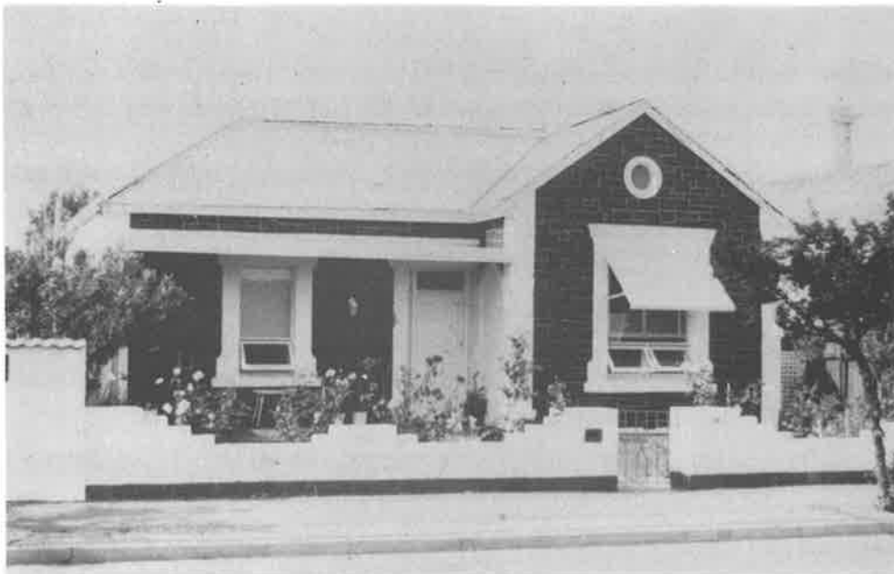
Plate 4.02. Plain Villa, built c 1900, Hyde Park; bluestone walls, galvanised iron roof.
