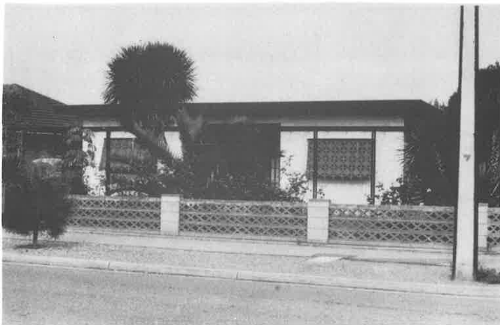
Plate 4.10. Contemporary, built 1950, Somerton Park; cement block walls, steel roof.
