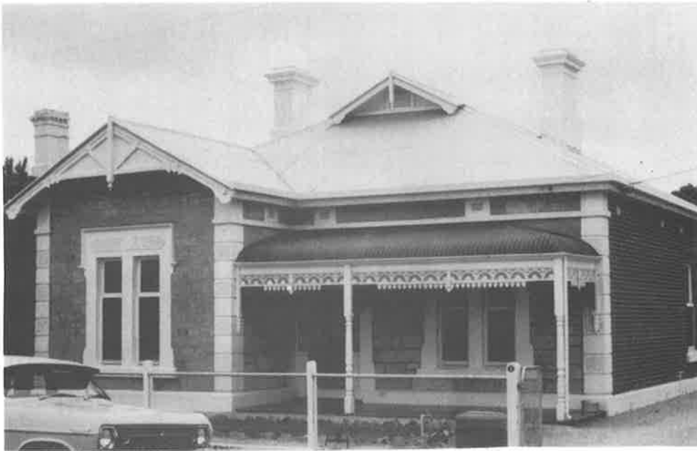
Plate 4.04. Louvred Roof Villa, built c 1905, Unley; red brick and freestone walls, galvanised iron roof.
