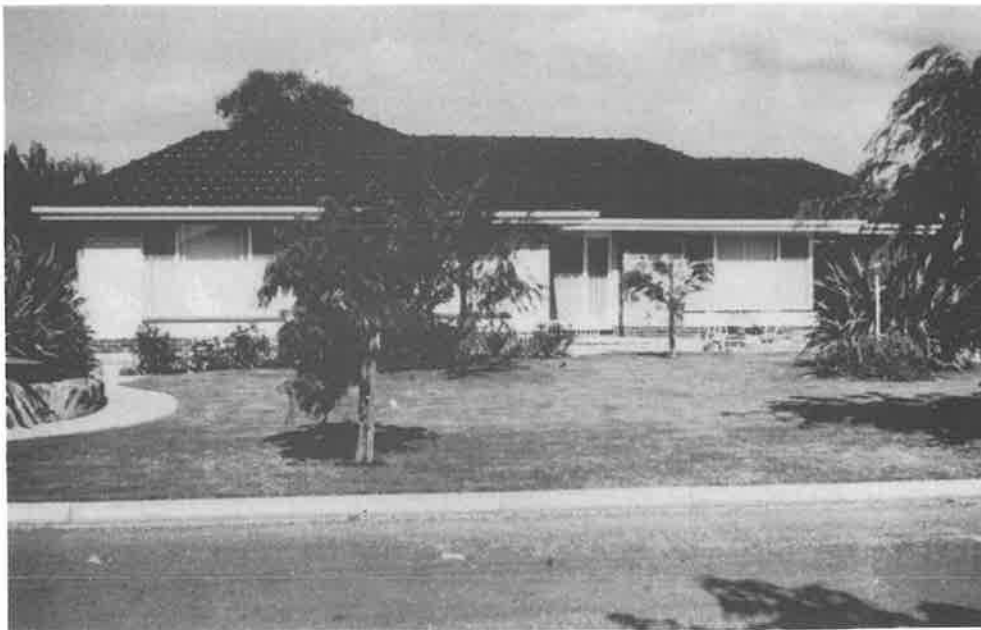
Plate 4.12. Triple-front, built 1968, Edwardstown; cream brick walls, black tiled roof.
