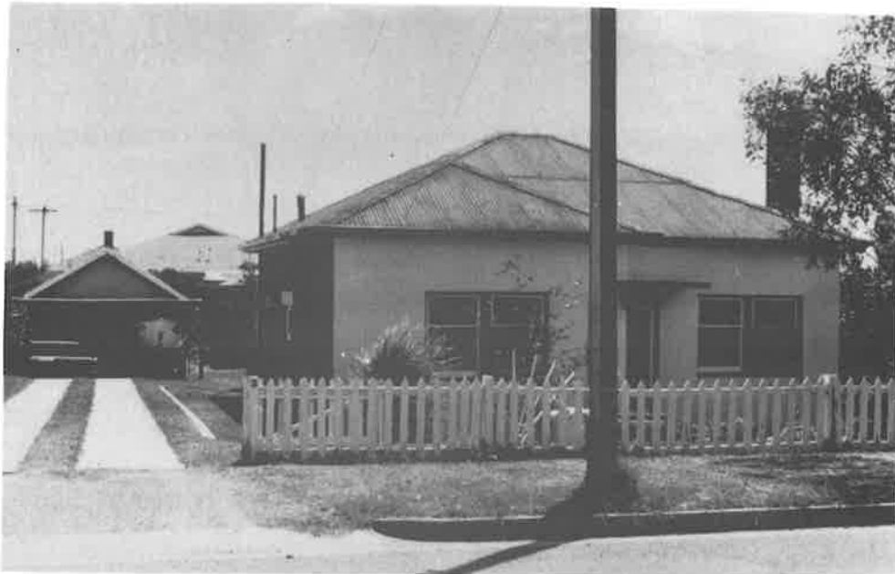
Plate 4.09. Austerity, built 1946, Somerton Park; red brick walls, galvanised iron roof.
