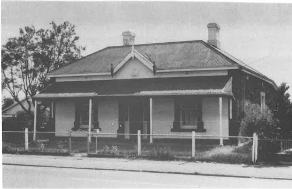
Plate 4.01. Symmetrical front, built c 1895, Clarence Park; bluestone walls, galvanised iron roof.
