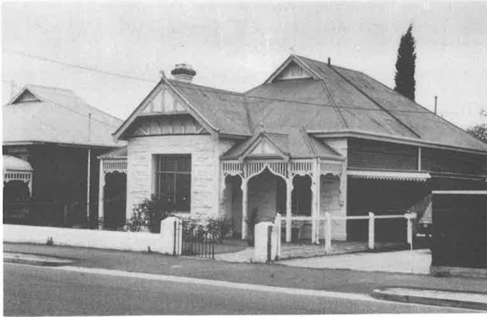
Plate 4.05. "Queen Anne", built c 1920, Hyde Park; red brick and sandstone walls, galvanised iron roof.
