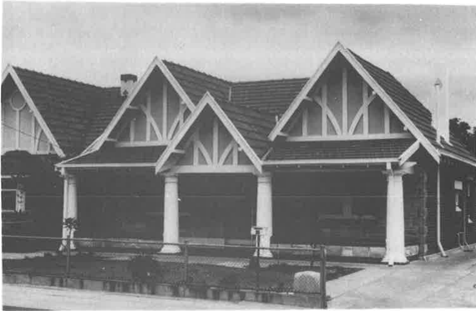
Plate 4.07. Tudor, built 1930, Unley; red brick and sandstone walls, tiled roof.
