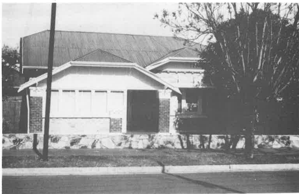
Plate 6.02. Enclosed front verandah on bungalow, built 1929; east-facing house.
