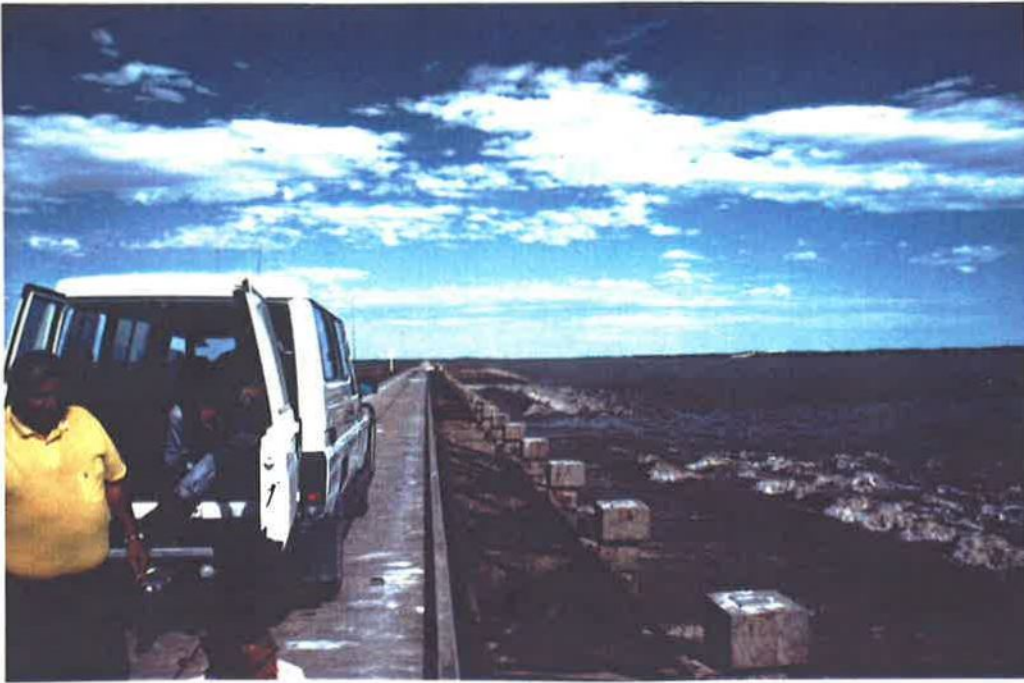
Fig.6.3 The barrages at Tauwitchere Island, 1993 (Photo: P.A. Clarke)
