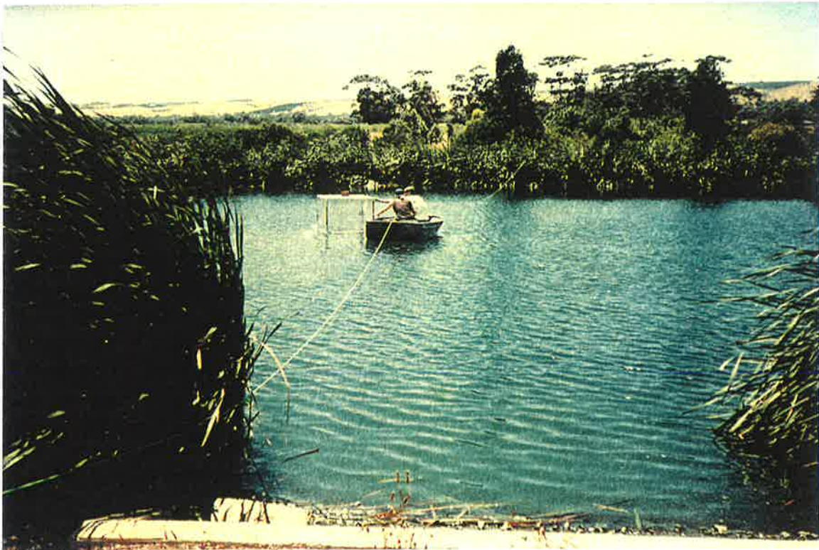
Figure 3.2: Willunga Wetlands, in the southern suburbs of Adelaide, a constructed wetland receiving secondary treated sewage effluent.
