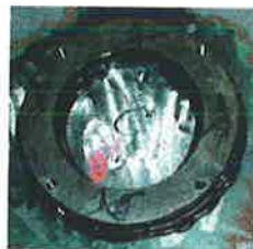
Figure 6.8: Mounting plate used to affix the AURA shaker onto the transformer.
