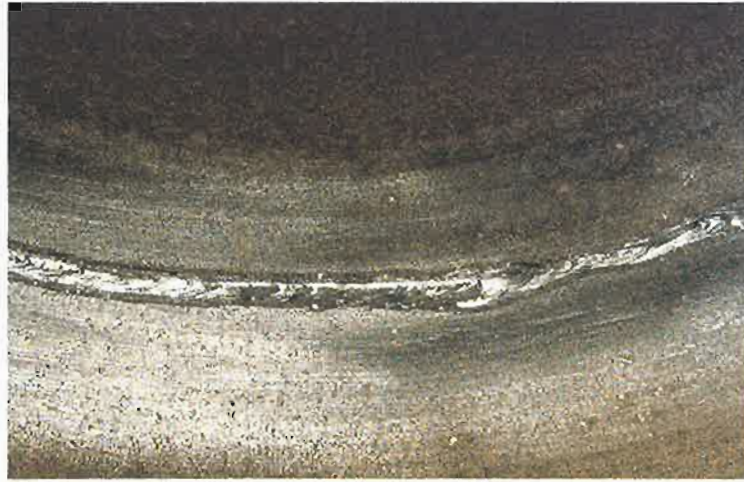
Figure 4.10: Inside pipe where residual stress measurements were made.
