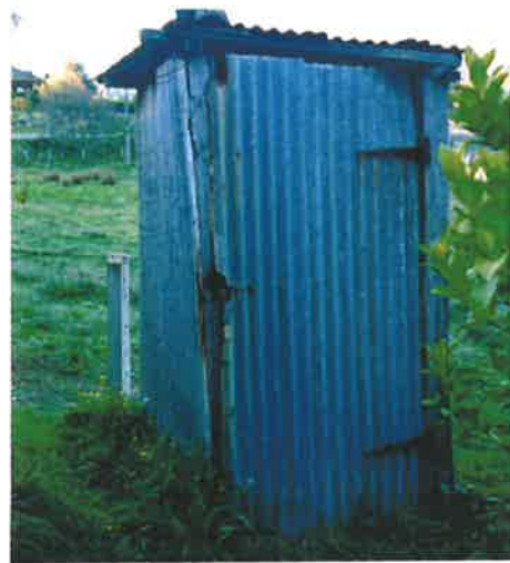
Corrugated iron smokehouse
